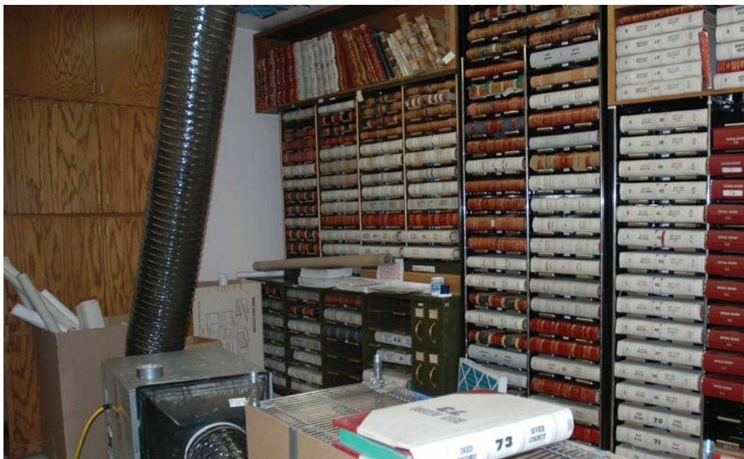
Record book storage vault with metal roller shelving; a temporary positive air ventilation system is set up to help with soot extraction. Photo credit: Randy Silverman
